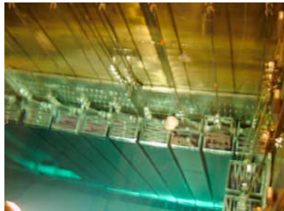
▲The Container Loaded with Compressed CRB Blades Hanged Inside the Spent Fuel Pool
