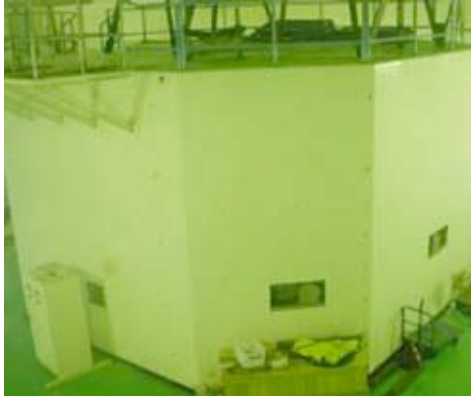
▲Before Dismantling of WBR Biological Shield in Building 019
