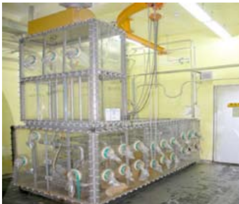
▲Unit 20 Glove Box in Building 016 Before Dismantling
