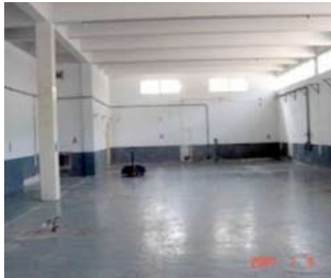
▲After Cleanup of Room 110 in Building 021
