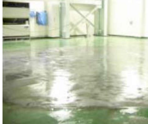
▲After Dismantling of WBR Biological Shield in Building 019
