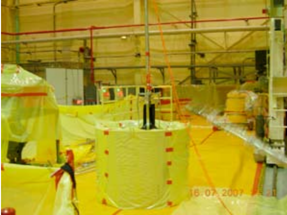
▲The Loading of CRB Velocity Limiter into the Waste Barrel
